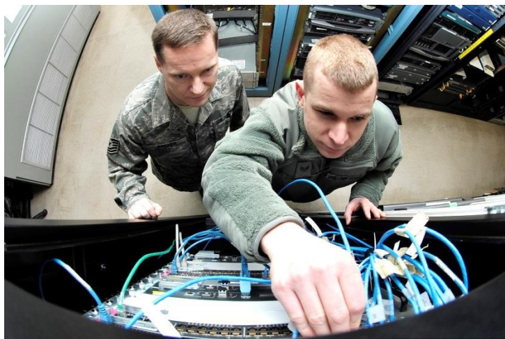
Air Force Tech Sgt. Kevin Garner and Air Force Senior Airman David Solnok, cyber transport technicians assigned to the 354 th Communications Squadron, hook cables in to the new Air Force Network router system at Eielson Air Force Base, AK. (U.S. Air Force photo by Staff Sgt. Christopher Boitz)
